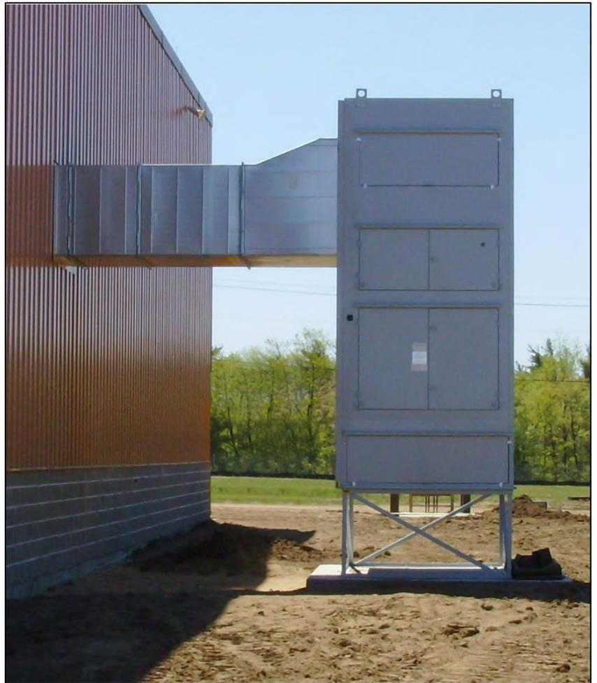
The **Heated Air Make-Up** is housed in a self-contained unit with latching hinged panel access to all filters, system components, and electrical controls.
